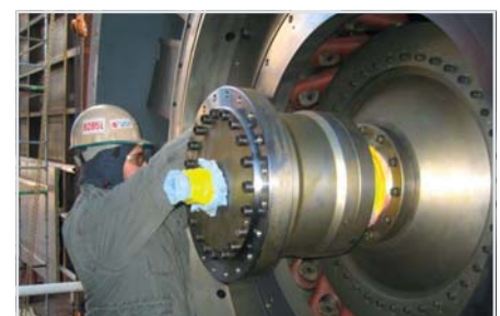
Mounting of the hydraulic cylinder.
