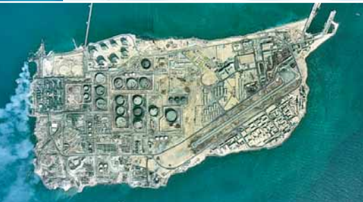
Gas liquefaction plant installed by ADGAS in DAS Island.
