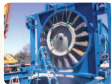
◀ Main Ventilation Fan During Installation
