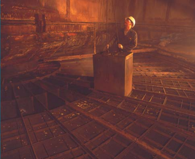
Removal of hot end element baskets.
