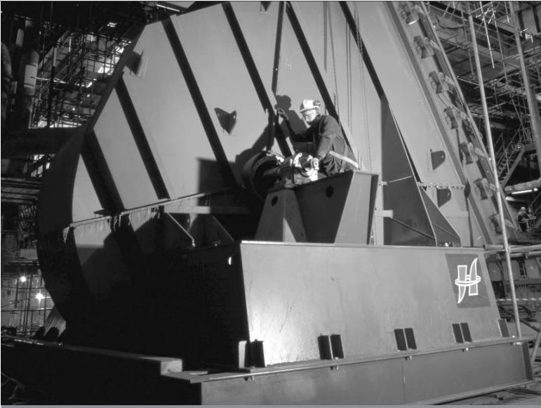
Gas recirculation fan being installed on the gas reburn system.
