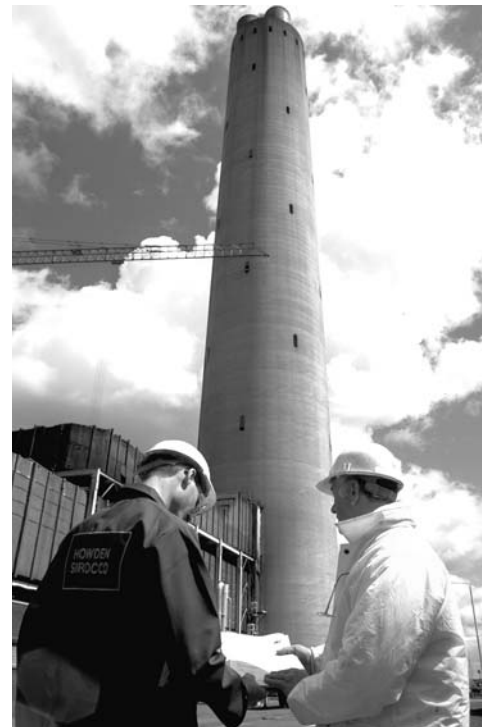
Howden engineers at site.
