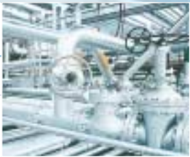
Pipe work: design manufacture & installation
