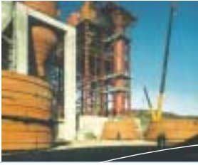
Complete turnkey plant construction & operation
